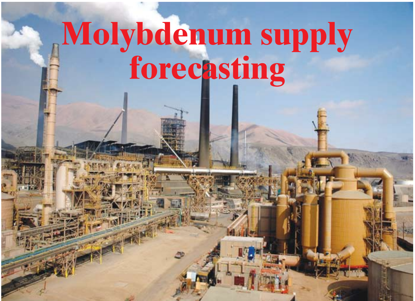
A new plant is pictured at the right, at Cujone Mine in southern Peru. At the end of the project, it will allow the mine to capture 95 percent of all emissions.
